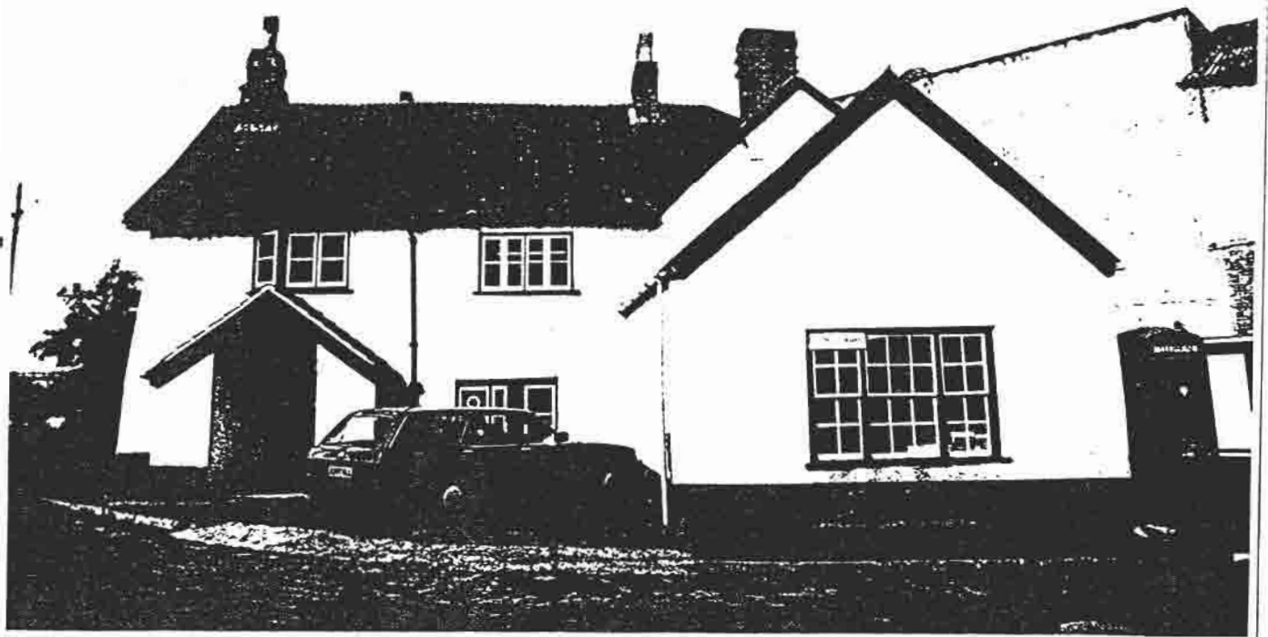
Figure 1. Silverton Mill; Cottage Office Block.
